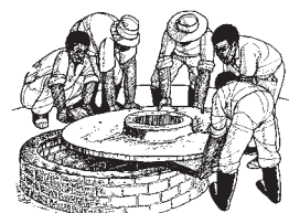
Set the well cover in place.
